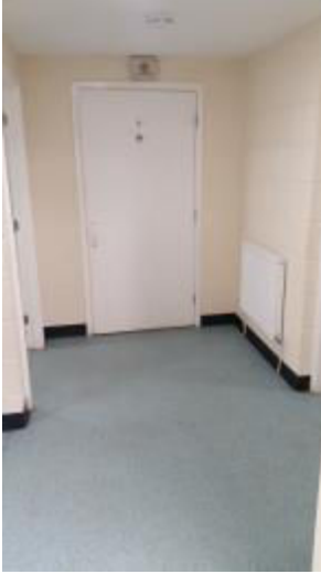
Disabled Toilet - External
